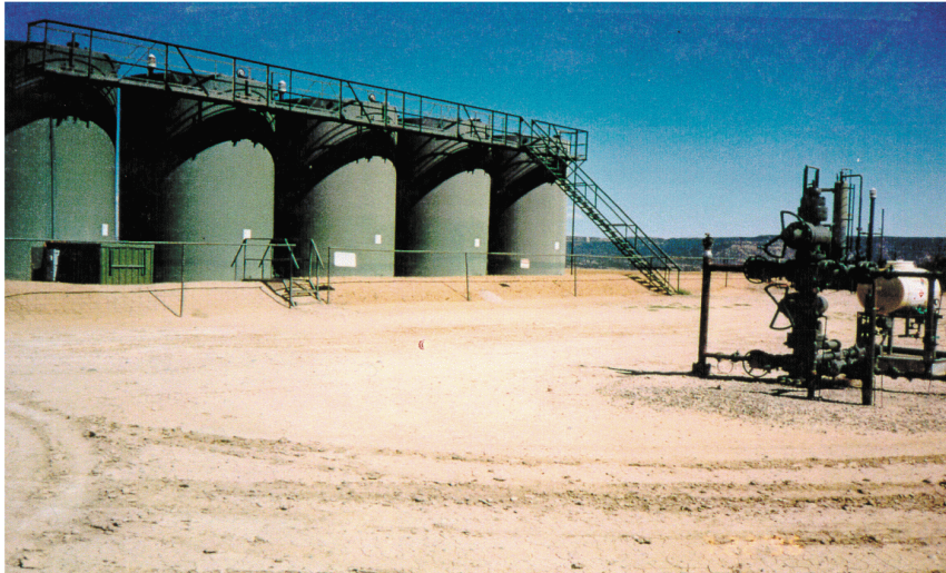
Photo 3-9 On-site Water Storage Tank
