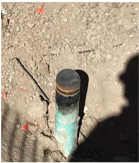
Cut/cap point at WTS – S end of line. Cut/Cap point is located at ~40" below final grade.
