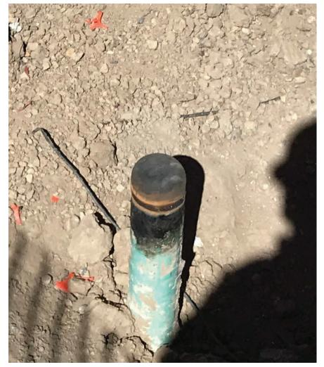
Cut/cap point near valve can – N end of line. Cut/Cap point is located at ~42" below final grade.
