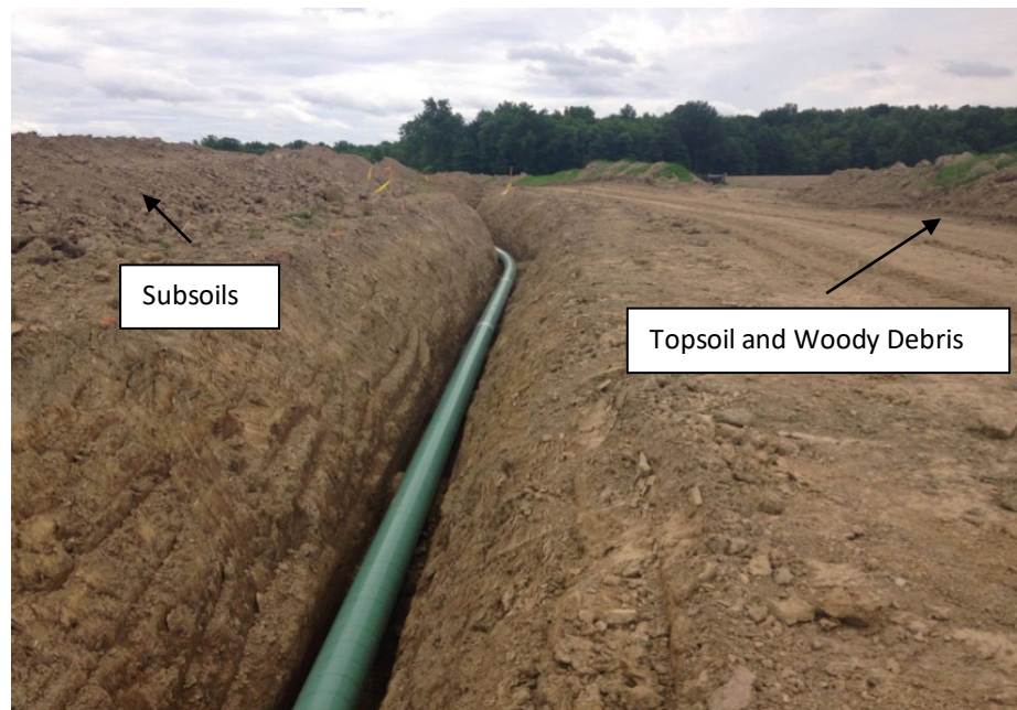
Figure 2. Example of a pipeline after trenching and placement.
