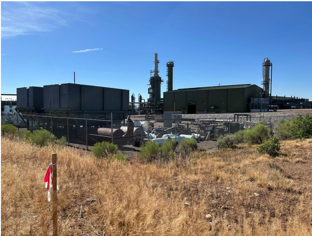
Photo 3. Looking east at adjacent existing facility and storage area.
